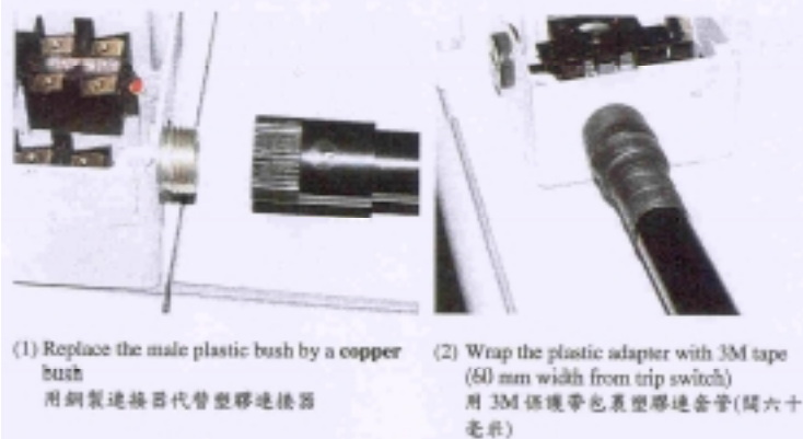
Photo 2 – TDI Trip Switch Conduit and Adapter (After Modification)
