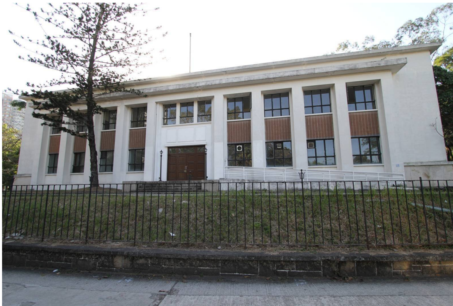
Photo of the existing Former Fanling Magistracy 前粉嶺裁判法院照片
