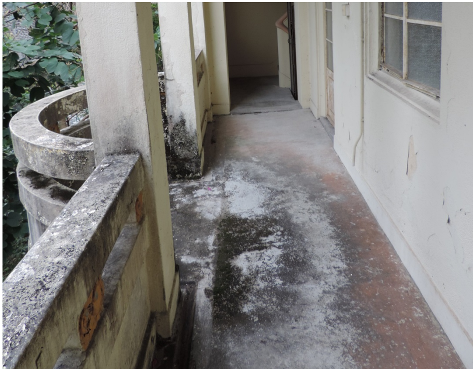
Corridor at the Servants' Quarters 工人宿舍走廊
