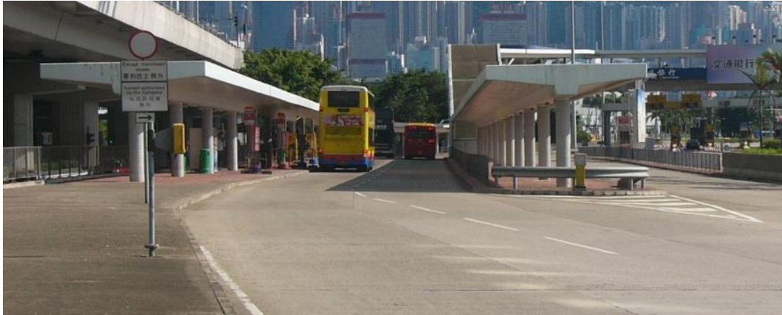
These rigid concrete bus stop canopies could destroy the entire upper deck of an errant double decker bus. Interim measures would include protocols requiring bus drivers to slow down as they exit from the high speed road
