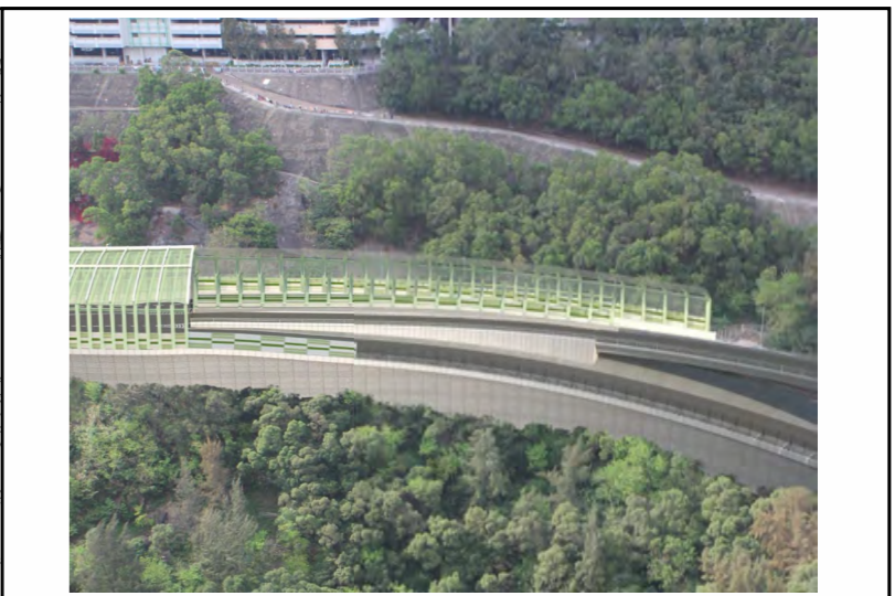
半開放式隔音罩及隔音屏障模擬照片 NOISE SEMI-ENCLOSURE AND NOISE BARRIER PHOTOMONTAGE
