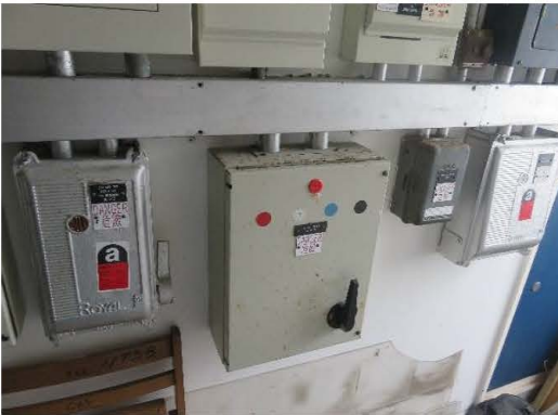
Photo 4581: Switch box with ACM containing arc cloth in Switch Room on the 5/F of CAS Headquarters
