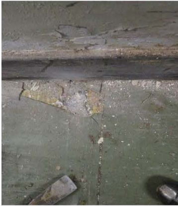
Photo 2221: Vinyl floor tile with mastic in store room on the G/F of EMSD Headquarters
