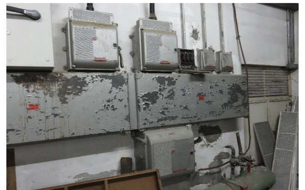
Photo 2136: Switch box with ACM containing arc cloth in Chiller Room on the roof of EMSD Headquarters
