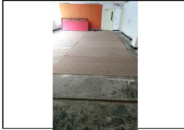
Photo 0007: Vinyl floor tile with mastic (ACM) in Officers' Mess on the 1/F of CAS Headquarters
