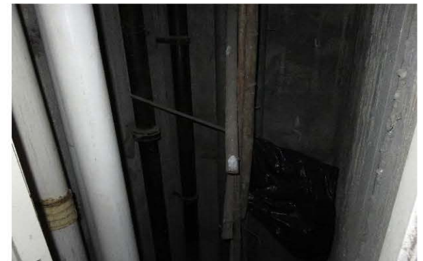
Photo 1940: Rain water and sewage pipes were made of PVC and cast iron in EMSD Headquarters
