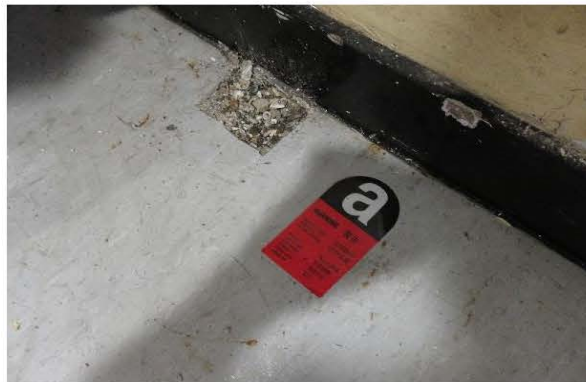
Photo 2209: Vinyl floor sheet with mastic (ACM) in cargo lift lobby on the 2/F of EMSD Headquarters
