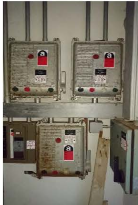
Photo.0082: Switch box with ACM containing arc cloth in Switch Room on the 6/F of CAS Headquarters
