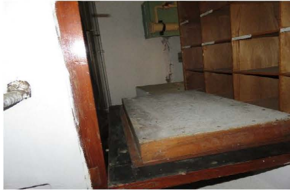
Photo 2463: Insulation board (ACM) inside heater box in A/C plant Room, 6/F, CAS Headquarters
