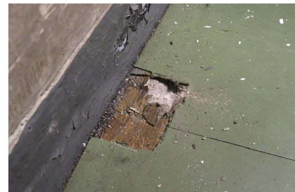
Photo 2212: Vinyl floor tile with mastic in cargo lift lobby on the 1/F EMSD Headquarters
