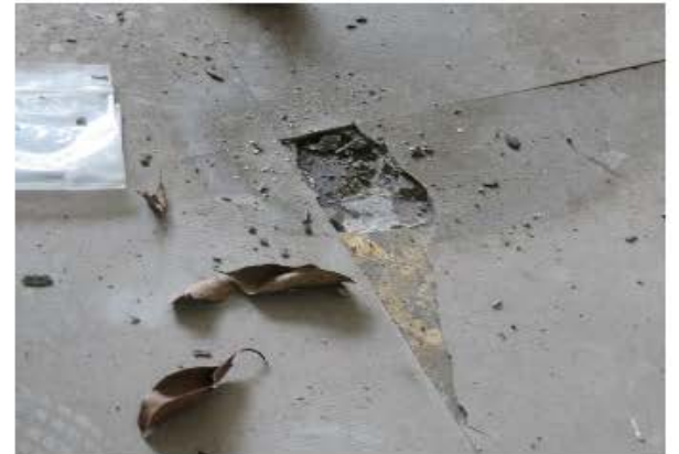
Photo 2427: S30, vinyl floor tile with mastic in living room of Room 1, 1/F, Quarter Block. ACM was identified. (Lab ID: B/103/16/30)
