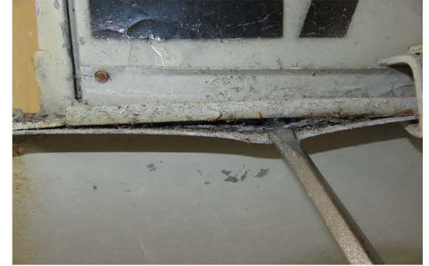
Photo 2066: No ACM flange gasket in the exhaust gas air-duct in E&M Workshop
