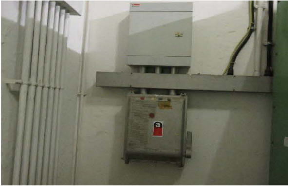
Photo 2483: Switch box with ACM containing arc cloth in Main Switch Room on the G/F of EMSD Headquarters
