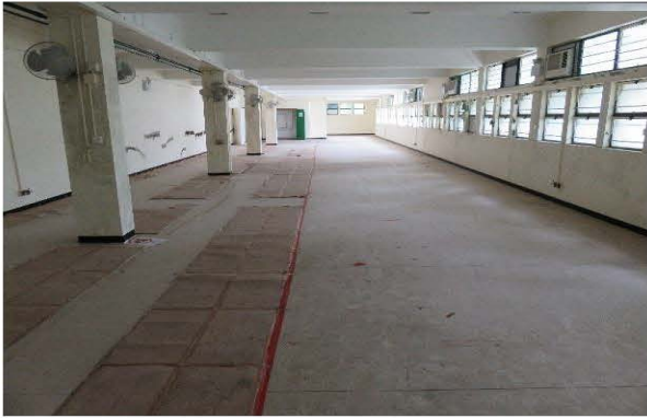
Photo 2346: Vinyl floor sheet with mastic (ACM) in office / workshop area on the 1/F of Training Centre
