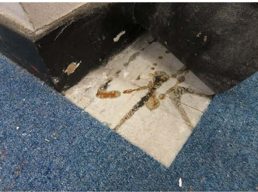
Photo 2515: Vinyl floor tile with mastic (ACM) in office area on the 1/F EMSD Headquarters
