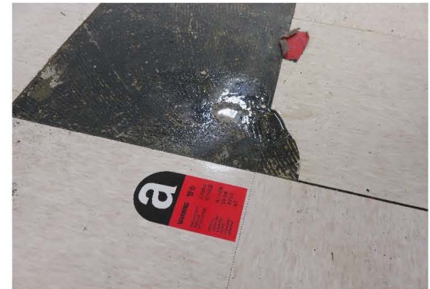
Photo 2180: S6, vinyl floor tile with mastic on 7/F, EMSD Headquarters. ACM was identified. (Lab ID: B/103/16/6)
