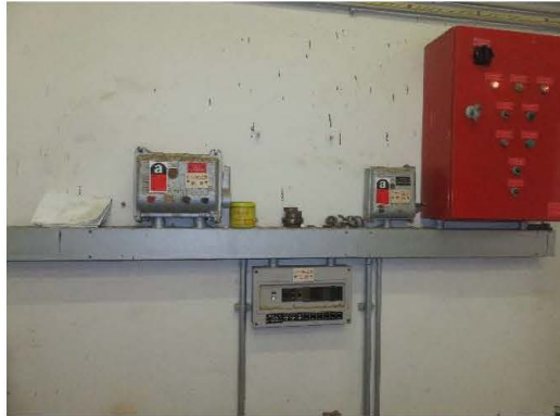
Photo 4584: Switch box with ACM containing arc cloth in Lift Machine Room on the Roof of CAS Headquarters
