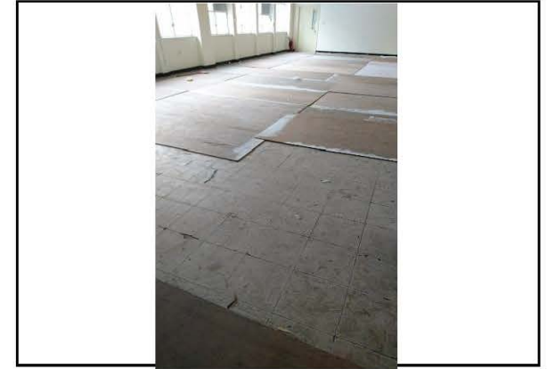
Photo 0009: Vinyl floor tile with mastic (ACM) in canteen on the 1/F of CAS Headquarters
