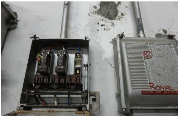
Photo 2133: Switch box with ACM containing arc cloth in Chiller Room on the roof of EMSD Headquarters
