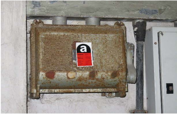
Photo 2369: Switch box with ACM containing arc cloth in Compressor Room on the G/F of Training Centre
