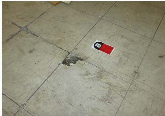
Photo 2459: S47, vinyl floor tile with mastic in CAS HQ canteen, 1/F, CAS Headquarters. ACM was identified. (Lab ID: B/103/16/47)
