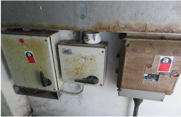
Photo 2378: Switch box with ACM containing arc cloth in Garage of the Workshop
