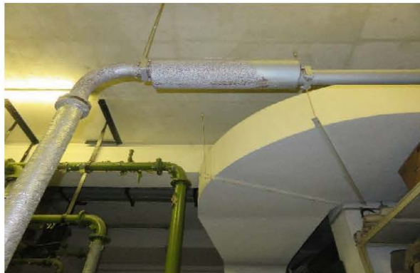
Photo 2477: Hard gasket at flue flange of generator in the 1st Basement, EMSD Headquarters
