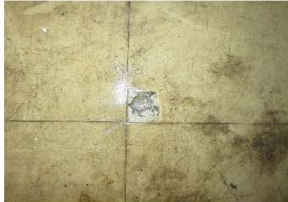
Photo 2425: S29, vinyl floor tile with mastic in Store Room of AMI Office, G/F, Quarter Block. No ACM was identified. (Lab ID: B/103/16/29)
