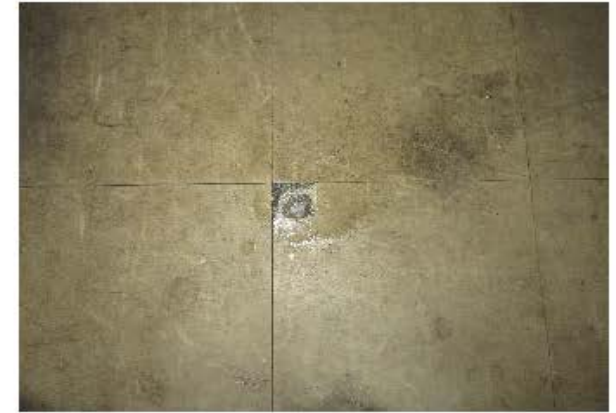
Photo 2423: S27, vinyl floor tile with mastic in TSCS Team Office, G/F, Quarter Block. No ACM was identified. (Lab ID: B/103/16/27)
