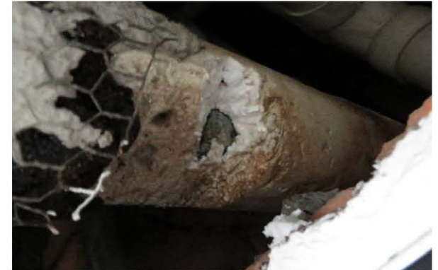
Photo 1869: Foam was identified in the chiller pipes of EMSD Headquarters
