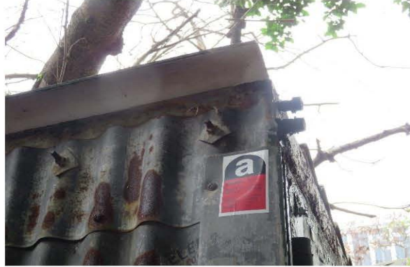
Photo 2445: Corrugated cement sheet roofing of DG Store, Workshop
