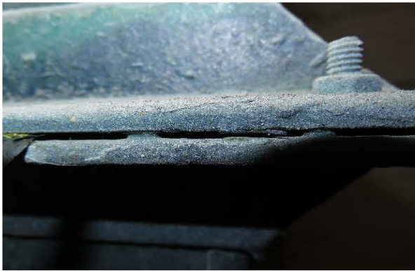
Photo 2080: No ACM flange gasket in the exhaust gas air-duct in E&M Workshop
