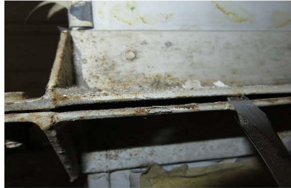
Photo 2082: No ACM flange gasket in the exhaust gas air-duct in E&M Workshop
