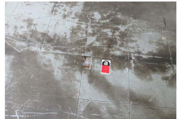
Photo 2454: S42, vinyl floor tile with mastic in Room G11, G/F, Training Centre. ACM was identified. (Lab ID: B/103/16/42)
