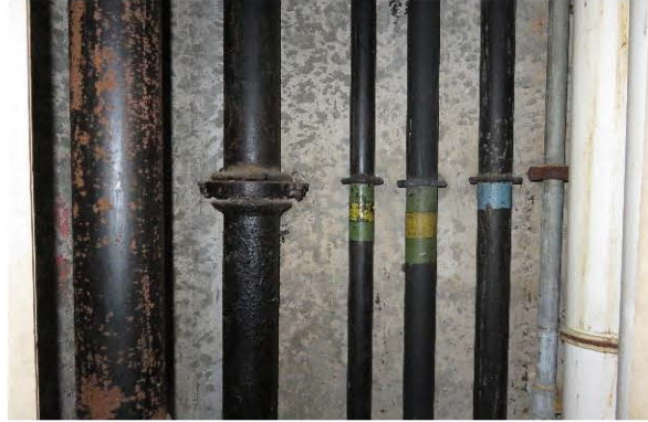
Photo 1867: Sewage pipes were made of cast iron in EMSD Headquarters
