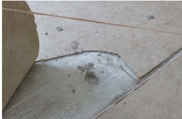
Photo 2295: Vinyl floor tile with mastic (ACM) in lift lobby on the 1/F of CAS Headquarters
