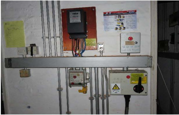
Photo 2138: Switch box with ACM containing arc cloth in Lift M/C & F/S Pumpo Room on the roof of EMSD Headquarters
