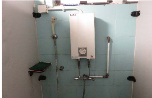
Photo 2098: Electrical hot water heater and hot water pipe with plastic lagging in male toilet in Post Office Recreation Club
