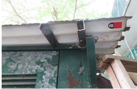
Photo 2370: Corrugated cement sheet on roof of a separate storage at the south-east to the Machine Shop in the Workshop
