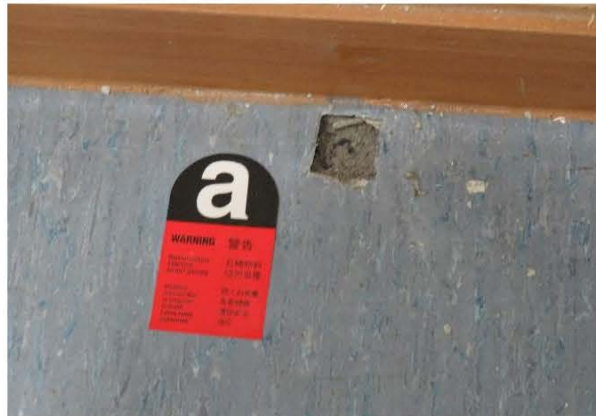
Photo 2177: S5, vinyl floor sheet with mastic in cargo lift lobby, 8/F, EMSD Headquarters. ACM was identified. (Lab ID: B/103/16/5)
