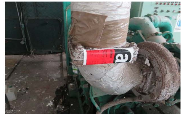
Photo 2435: Hard gasket at flue flange of generator in the Workshop
