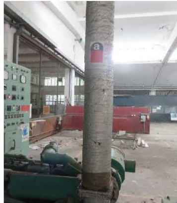
Photo 2434: Rope lagging on flue of generator in the Workshop
