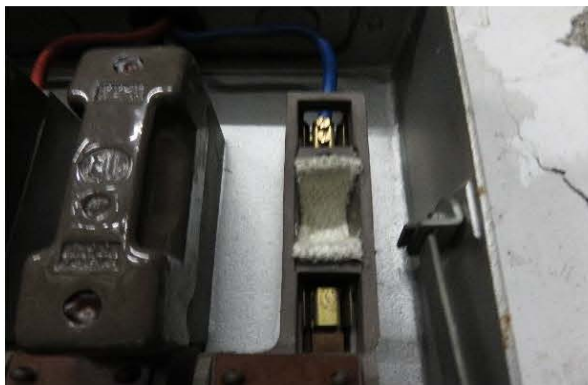
Photo 2135: Switch box with ACM containing arc cloth in Chiller Room on the roof of EMSD Headquarters
