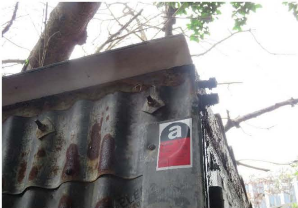
Photo 2445: S40, corrugated cement sheet at roof sheeting of DG Store, EMSD Workshop. ACM was identified. (Lab ID: B/103/16/40)
