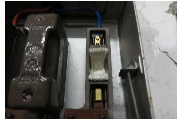
Photo 2135: S24, Arc cloth inside switch box in Chiller Plant Room, R/F, EMSD Headquarters. ACM was identified. (Lab ID: B/103/16/24)
