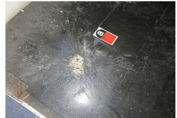
Photo 2462: S48, vinyl floor tile with mastic in Hall, 6/F, CAS Headquarters. ACM was identified. (Lab ID: B/103/16/48)
