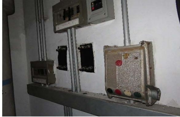
Photo 2139: Switch box with ACM containing arc cloth in Lift M/C & F/S Pumpo Room on the roof of EMSD Headquarters
