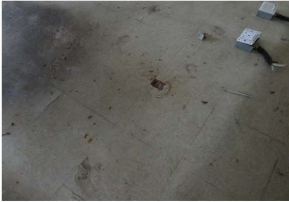
Photo 2438: S37, vinyl floor tile with mastic in Room G07, EMSD Workshop. No ACM was identified. (Lab ID: B/103/16/37)
