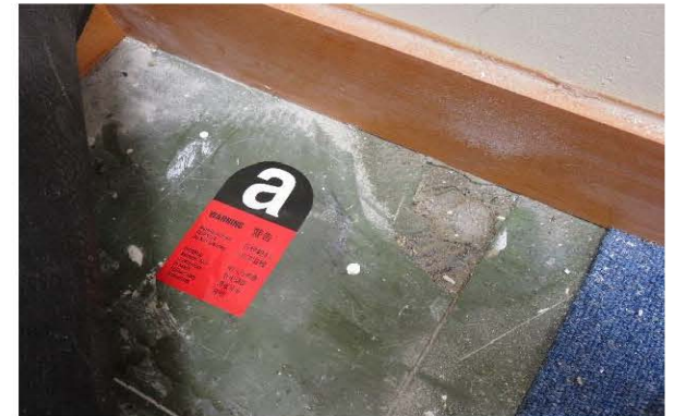
Photo 2175: Vinyl floor tile with mastic (ACM) in office area , 9/F, EMSD Headquarters
