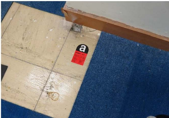
Photo 2173: S4, vinyl floor tile with mastic below floor mat on 8/F, EMSD Headquarters. ACM was identified. (Lab ID: B/103/16/4)
