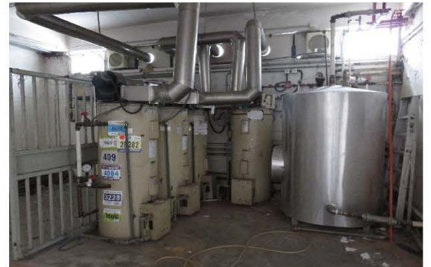
Photo 2055: Towergas hot water boilers at the bath room in E&M Workshop
