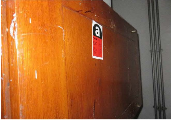
Photo 2467: S49, insulation board inside heater box in A/C plant Room, 6/F, CAS Headquarters. ACM was identified. (Lab ID: B/103/16/49)
