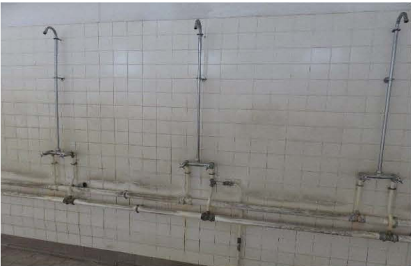
Photo 2049: Copper hot water pipes with PVC lagging in E&M Workshop
