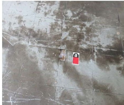
Photo 2454: Vinyl floor tile with mastic (ACM) in Room G11 on the G/F of Training Centre
