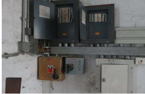
Photo 2379: Switch box with ACM containing arc cloth in Block C of the Workshop
