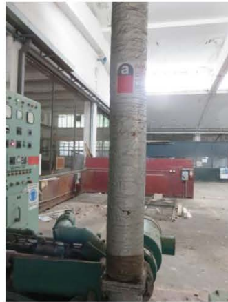
Photo 2434: S35, rope lagging on flue of generator, EMSD Workshop. ACM was identified. (Lab ID: B/103/16/35)
