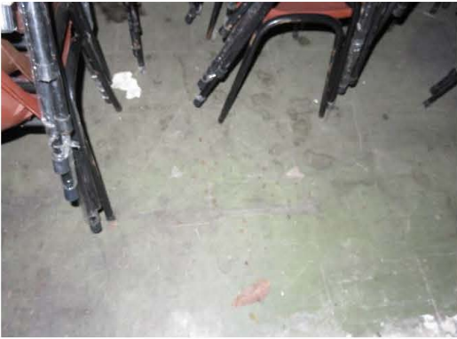
Photo 2519: Vinyl floor tile with mastic (ACM) in store room on the G/F of EMSD Headquarters
