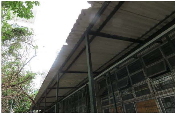
Photo 2372: Corrugated cement sheet roofing at the south-east to the Rooms G01, G02, G03, G05 & G06 in the Workshop
