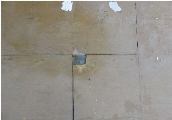
Photo 2433: S34, vinyl floor tile with mastic in living room of Room 12, 5/F, Quarter Block. No ACM was identified. (Lab ID: B/103/16/34)
