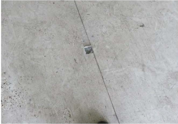
Photo 2455: S43, vinyl floor sheet with mastic on 1/F, Training Centre. No ACM was identified. (Lab ID: B/103/16/43)
