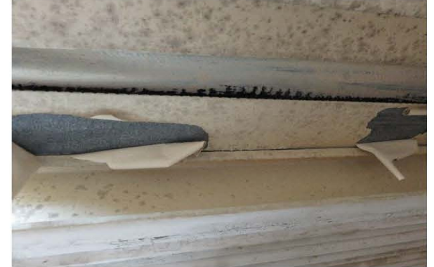
Photo 2104: Black plastic flexible joint for the air-duct inactivity room one in Post Office Recreation Club
