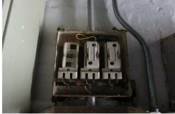
Photo 2490: Switch box with ACM containing arc cloth in A/C Plant & Store Room in the 1st Basement of EMSD Headquarters
