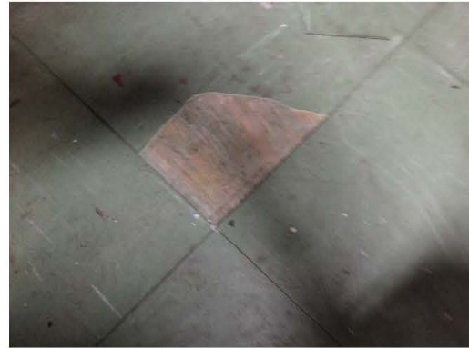
Photo 2516: Vinyl floor tile with mastic (ACM) in cargo lift lobby on the 1/F EMSD Headquarters
