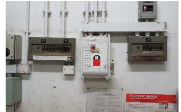
Photo 2482: Switch box with ACM containing arc cloth in Main Switch Room on the G/F of EMSD Headquarters
