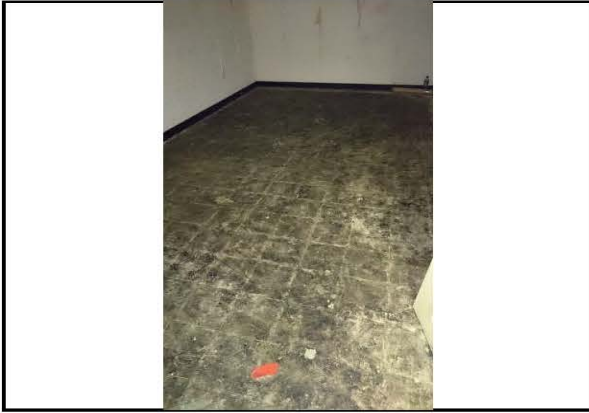
Photo 0006: Vinyl floor tile with mastic (ACM) in Game Room on the 1/F of CAS Headquarters
