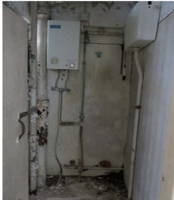
Photo 2329: Electrical hot water heater and hot water pipe with metal lagging in bathroom, 4/F, Quarter Block
