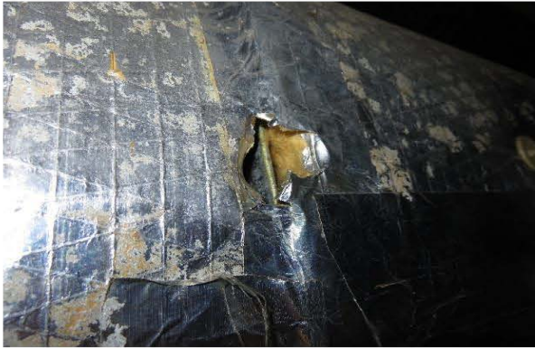
Photo 2092: No airduct gasket at the air-duct above activity room 3 in Post Office Recreation Club
