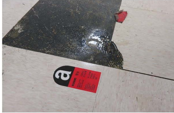
Photo 2180: Vinyl floor tile with mastic (ACM) in office area, 7/F, EMSD Headquarters
