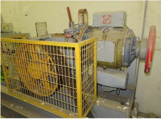
Photo 4586: Lift brake pad/shoe in Lift Machine Room on the Roof of CAS Headquarters
