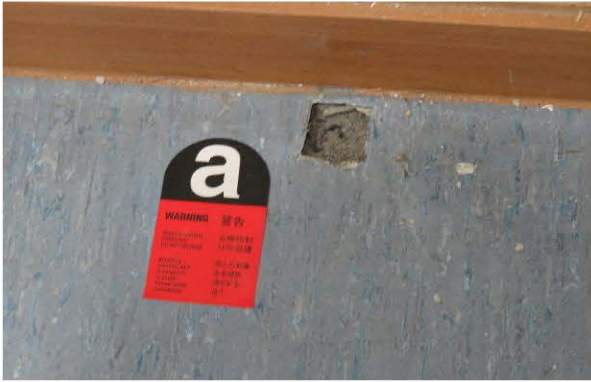
Photo 2177: Vinyl floor sheet with mastic (ACM) in cargo lift lobby on the 8/F of EMSD Headquarters
