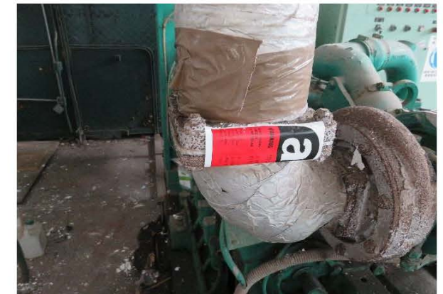
Photo 2435: S36, hard gasket at flue flange of generator, EMSD Workshop. ACM was identified. (Lab ID: B/103/16/36)
