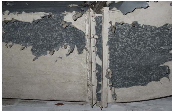
Photo 2376: No ACM air duct flange gaskets was identified in the Workshop
