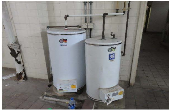
Photo 2053: Electrical hot water boilers at the bath room in E&M Workshop
