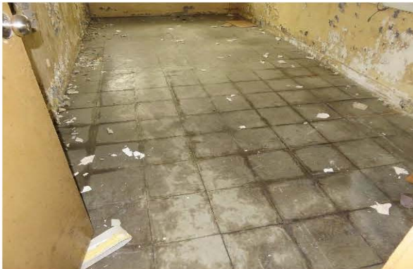
Photo 2366: Vinyl floor tile with mastic (ACM) in Room G11 on the G/F of Training Centre
