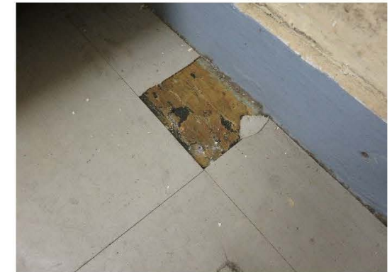
Photo 2518: Vinyl floor tile with mastic (ACM) in store room on the G/F of EMSD Headquarters
