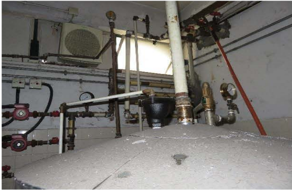
Photo 2056: Copper hot water pipes in E&M Workshop
