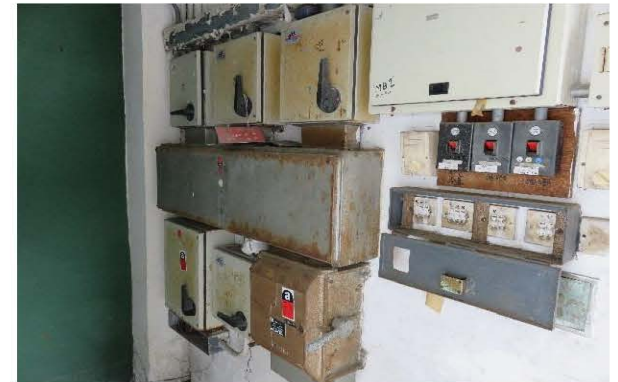
Photo 2377: Switch box with ACM containing arc cloth in Garage of the Workshop
