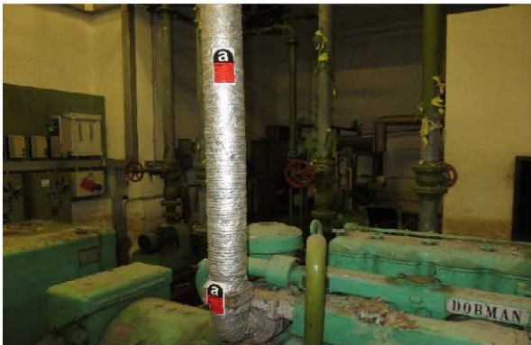
Photo 2476: Rope lagging on flue of generator in the 1st Basement, EMSD Headquarters
