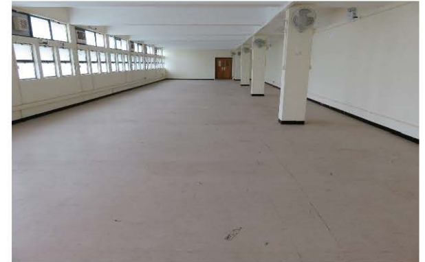
Photo 2359: Vinyl floor sheet with mastic (ACM) in office / workshop area on the 3/F of Training Centre
