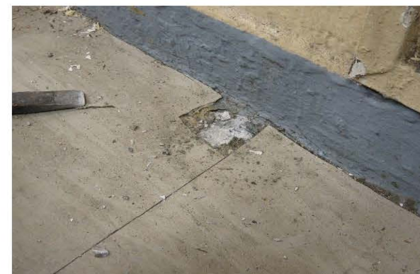
Photo 2219: Vinyl floor tile with mastic in store room on the G/F of EMSD Headquarters
