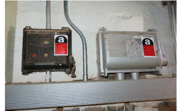
Photo 2491: Switch box with ACM containing arc cloth in A/C Plant & Store Room in the 1st Basement of EMSD Headquarters
