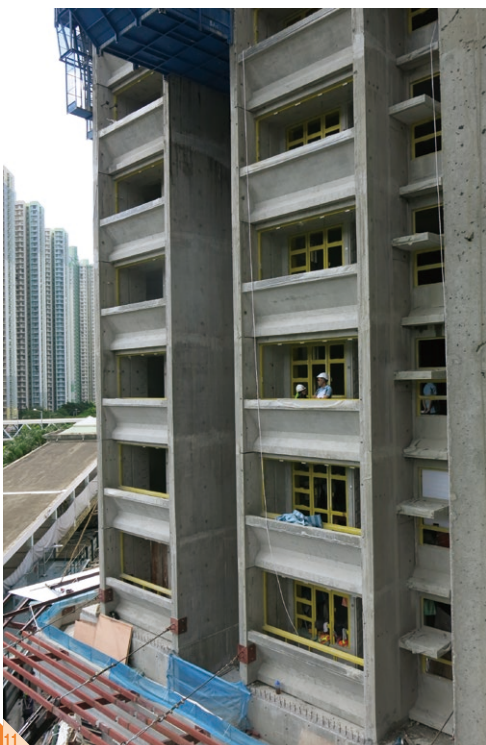
11 Acoustic balcony under construction (left) and its precast component
