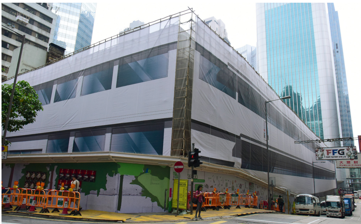
Central Market is now at advance works stage, mainly working at the areas near Queen's Road Central, which will become a new entrance plaza as part of the public open space.
