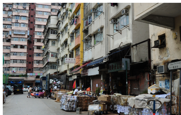
The dead-end of Chun Tin Street is included in the new KC-008(A) development scheme for pedestrian and traffic flow improvement.
