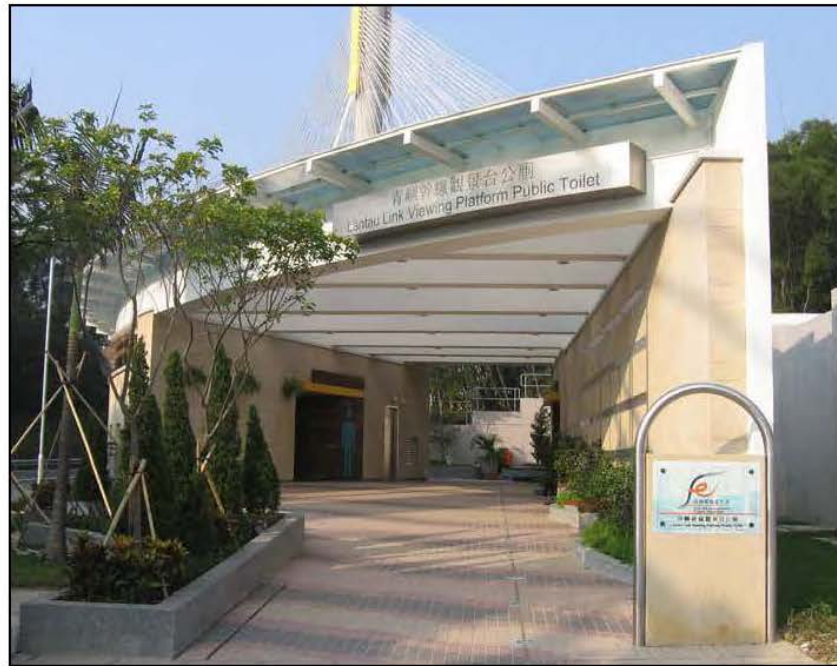
Lantau Link Viewing Platform Public Toilet (Kwai Tsing)
