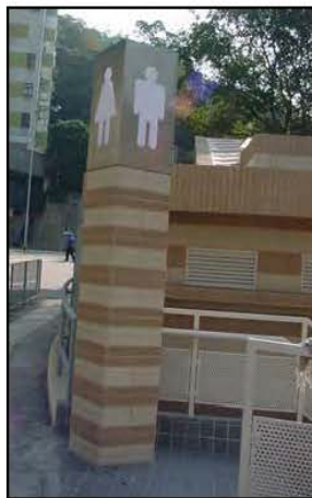
Tai Hang Road Public Toilet (Wanchai)
