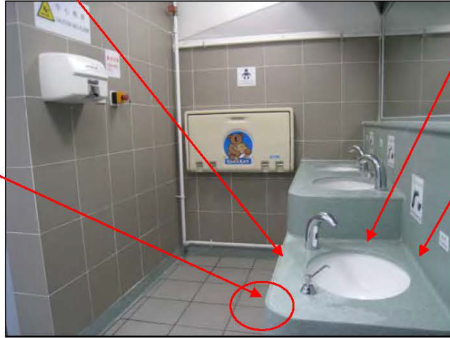
Kin Lung Street Public Toilet (Tuen Mun)
