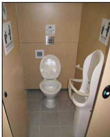
Baby rest (floor standing type with fixed front guard) in pedestal cubicle
