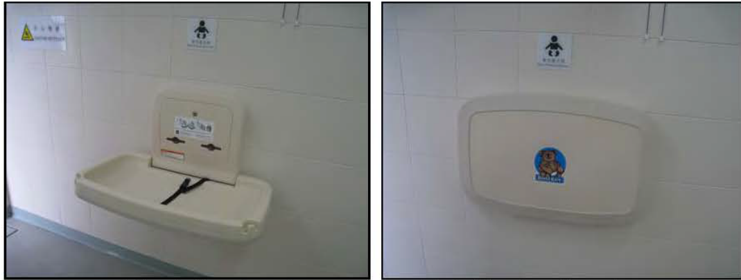
Folding baby changing counter with indicative sign above
