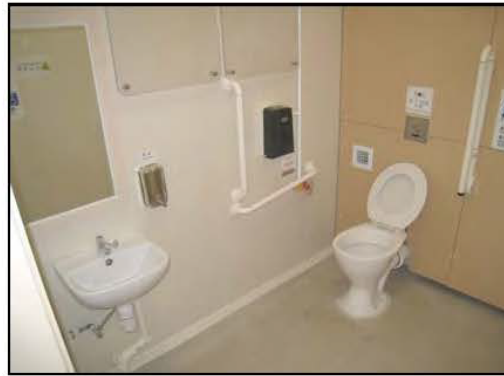
Tai Po Centre Public Toilet (Tai Po)
