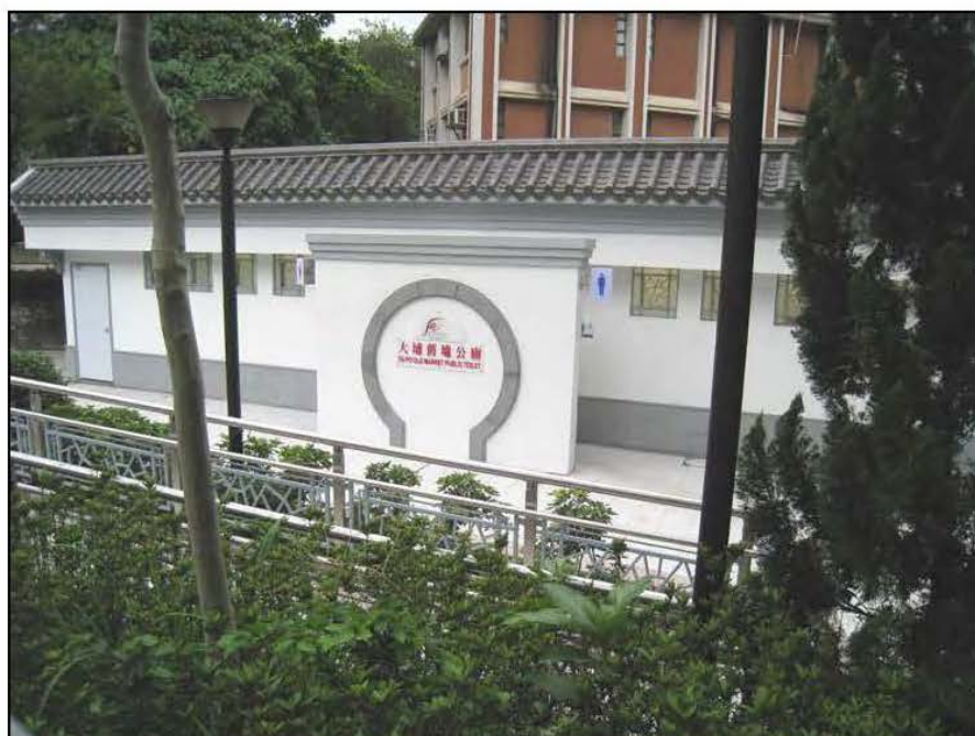
Tai Po Old Market Public Toilet (Tai Po)
