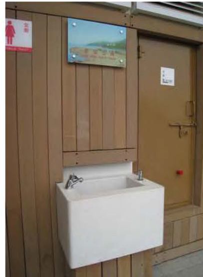
Wash hand trough outside the toilet premises
