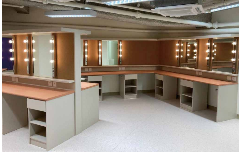
Renovation of four dressing rooms has been completed in August 2020. 四個化妝間在 2020 年 8 月完成裝修。
