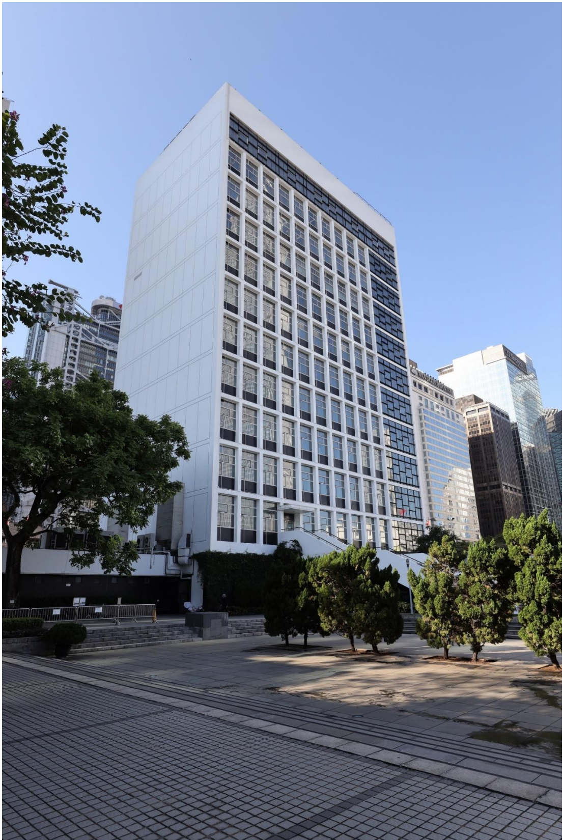
The north façade of High Block with “an uncomplicated repetitive fenestration in a concrete frame”; while the east façade is plastered white.
