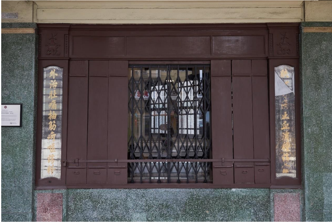
Shop windows with original window shutters facing Lai Chi Kok Road are retained.
