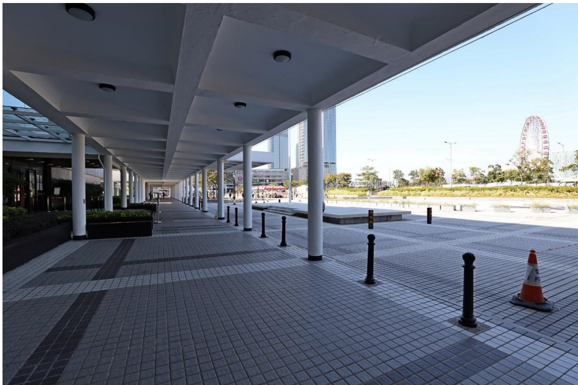
A covered walkway connecting Low Block, Memorial Garden and High Block.
