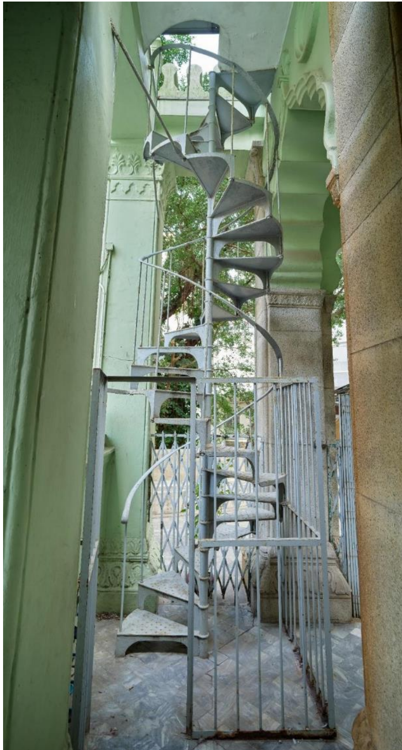
Metal spiral staircase at the corner of the entrance portico leading up to the minaret.
