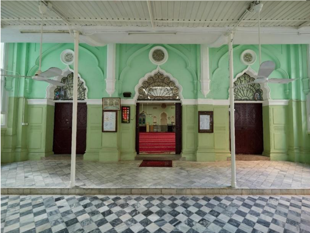
Three pointed multifoil archways at the entrance portico of the prayer hall. The floor of the entrance portico is finished with marble floor tiles.
