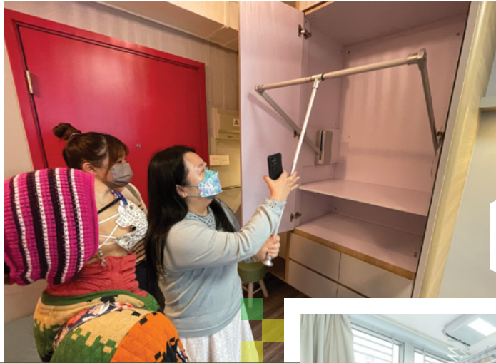
▲ Under the Home Improvement Community Programme, pull down rails are designed to facilitate elderly tenants' access to high hanging clothes in their wardrobes.
