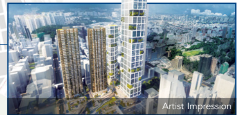
A comprehensive mixed-use development serving as a converging point of at-grade character streets, elevated walkways and nearby MTR stations
