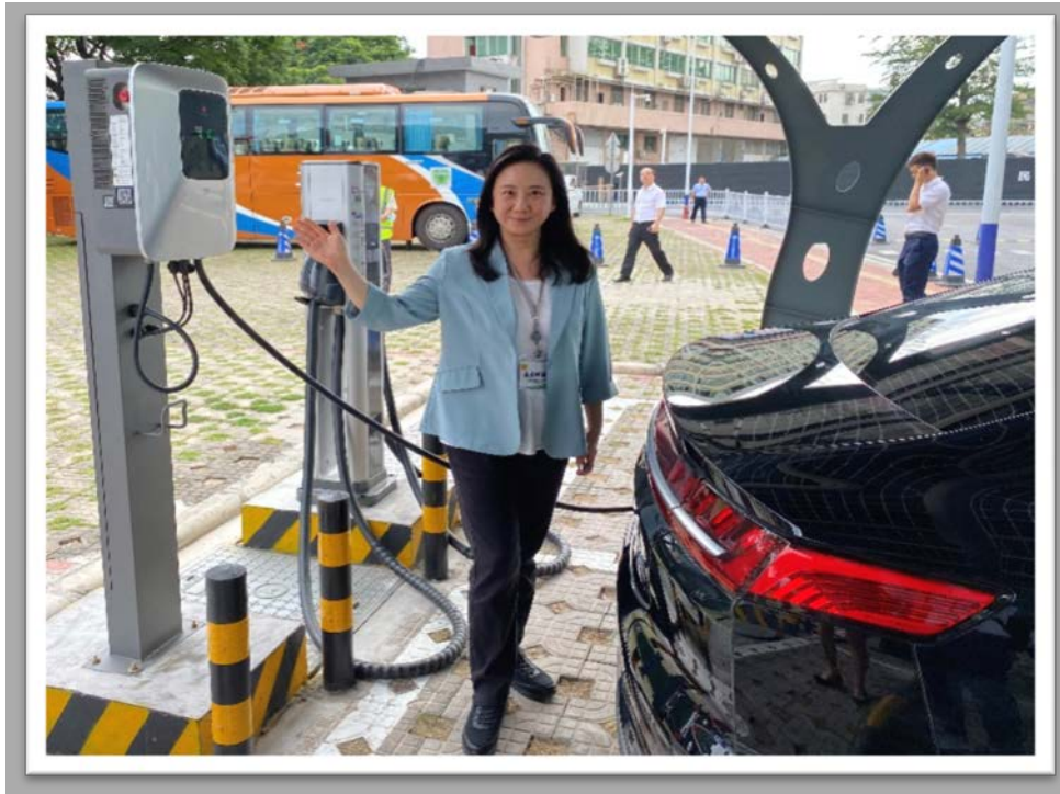
Leader of the Delegation, Hon Elizabeth QUAT, stands beside a charging post that supports “vehicle to grid” technique
