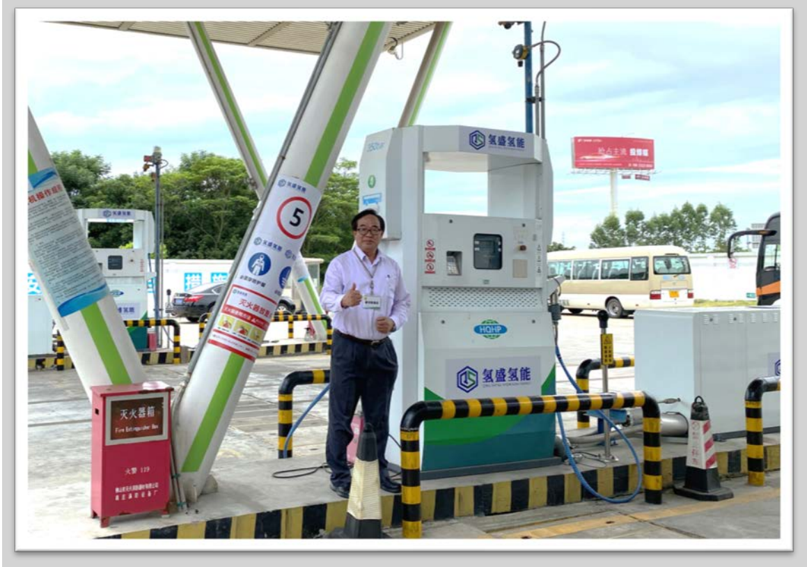
The hydrogen refueling service centre in Gaoming District, Foshan
