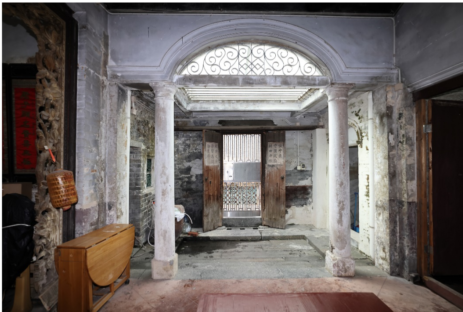
Light well right behind the main entrance with Tuscan columns and arch
