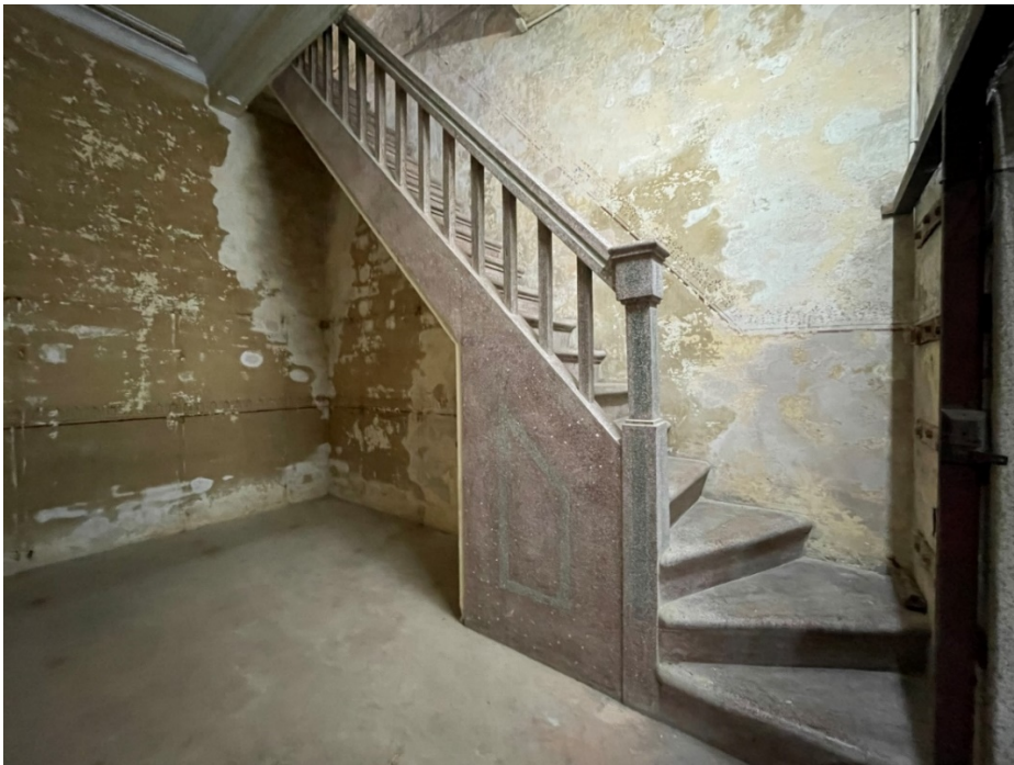
Staircase finished in red and green terrazzo inside the watchtower
