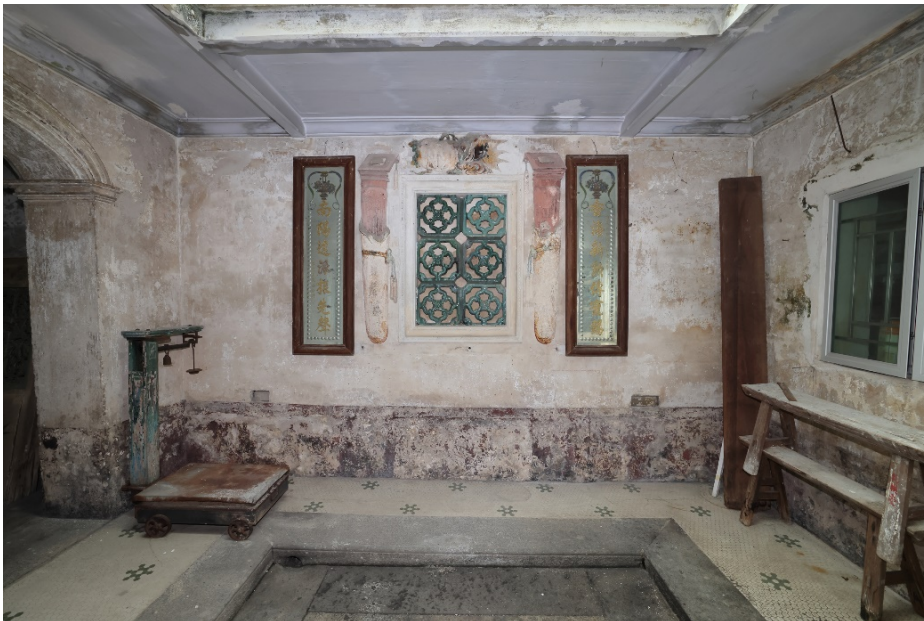
Green glazed ceramic grilles topped by a plaster moulding of auspicious motif
