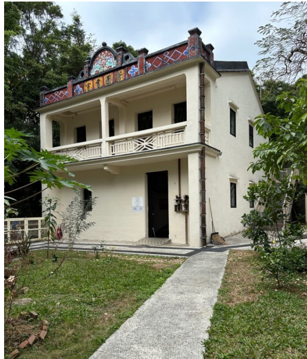
Existing Condition of FYSH 芳園書室的現貌
