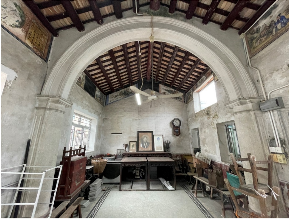
Tuscan columns and arch in the new study room
