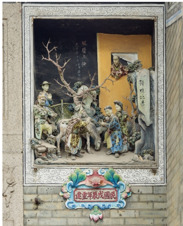
Colourful plaster moulding figurines at the front façade
