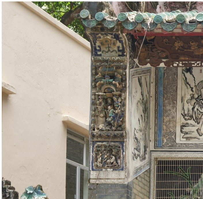
Chitou (gable wall head) decorated with ceramic figurines at the front façade
