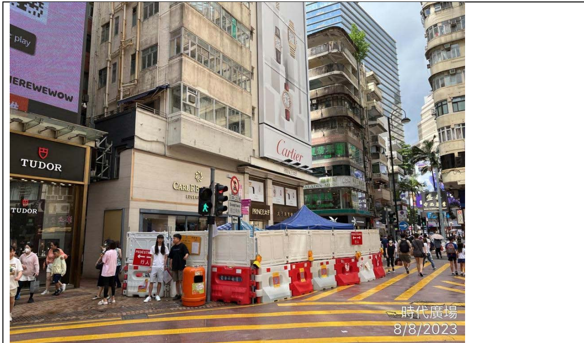
Traffic diversion or road closure at busy road junction
