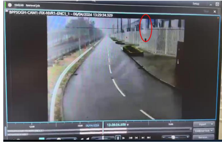
Figure 4 Lightning Observed at the Vicinity of C6 Generator Transformer Compound around 3 seconds prior to Discharge at C6
