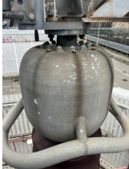
Figure 14 Patches of Metal on C6 Connector Head
