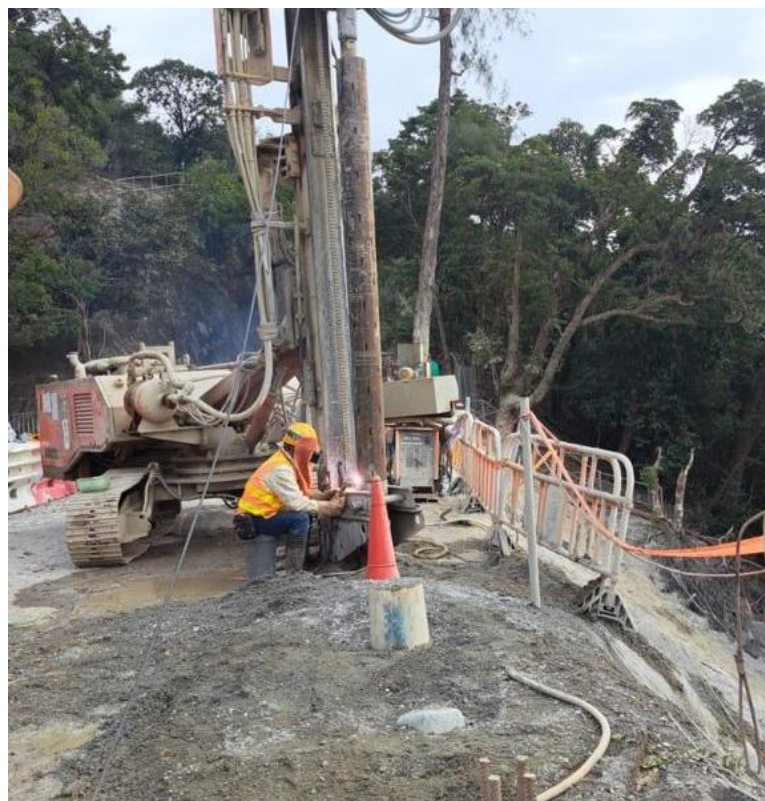
Installation of mini-piles to stabilise the slope
