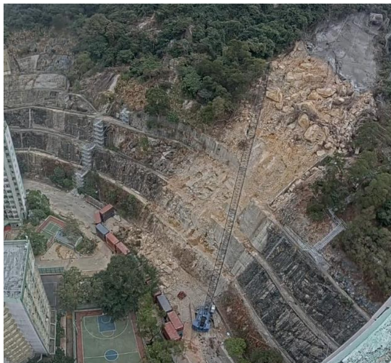
Using large crane to remove debris from the slope surface
