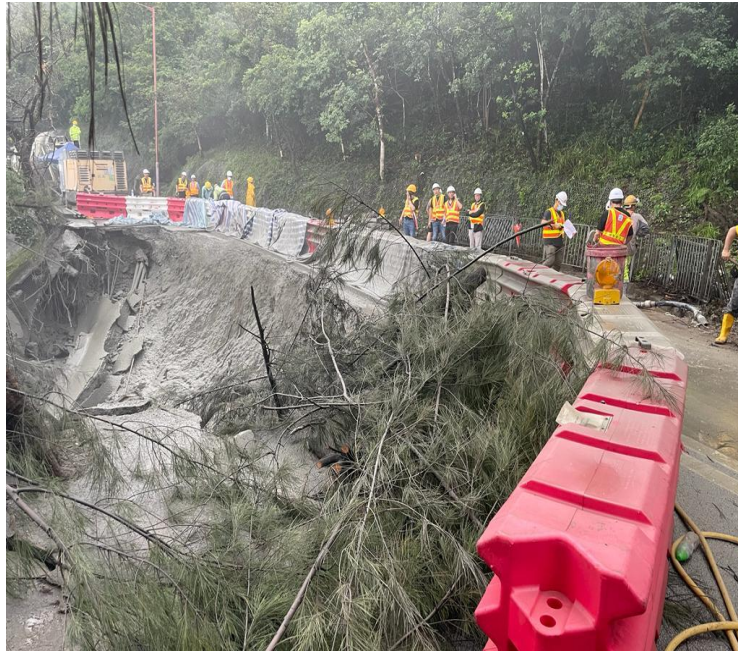
Shotcreting to stabilise the location of the landslide
